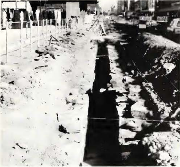
Fig. 1. The water furrow during excavation.
